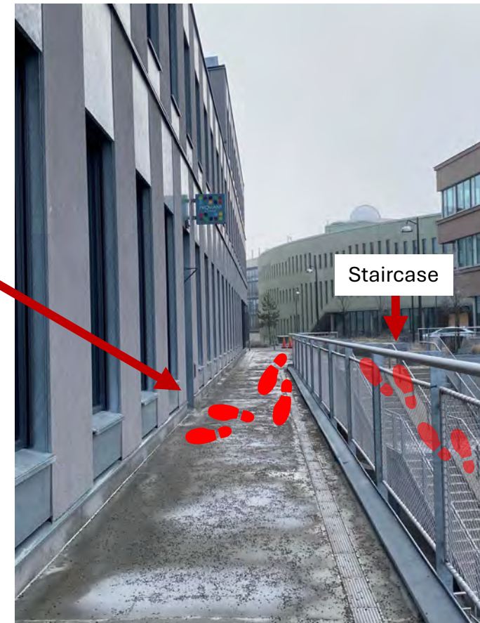
Close-up photo of the Proviant entrance
